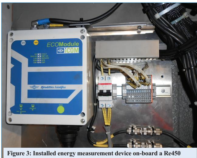
**Figure 3: Installed energy measurement device on-board a Re450**
